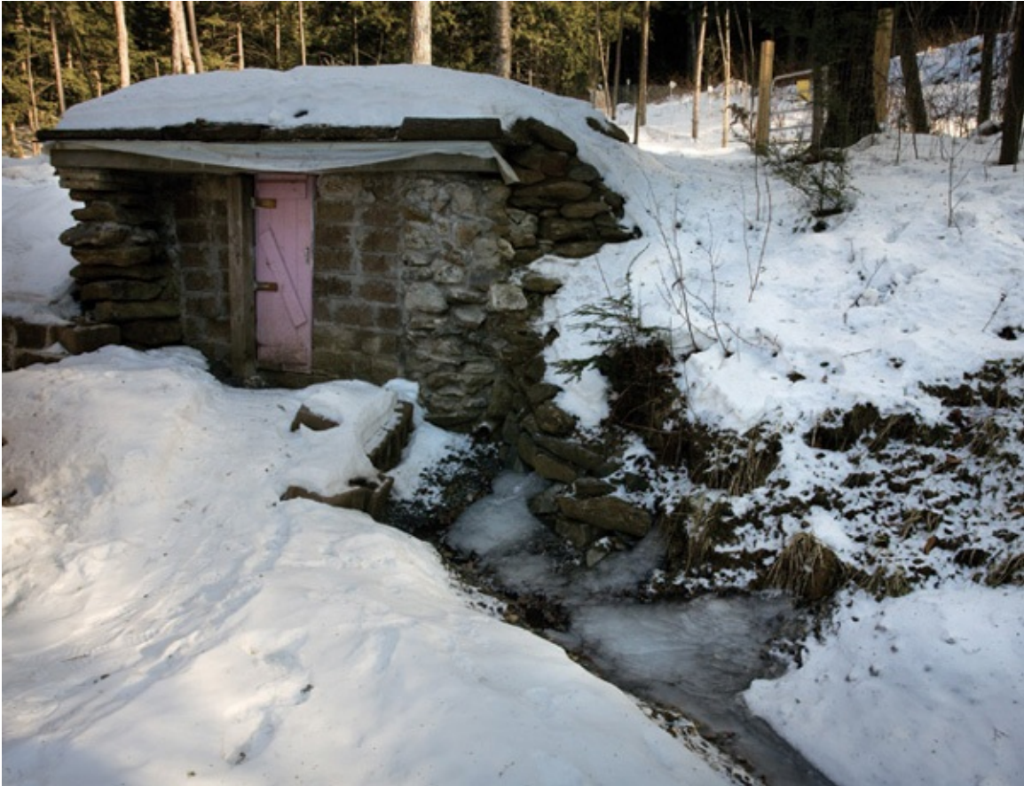
Built into a hillside at True 4 Now Farm in the root cellar is a cooler space than the ground-floor bathroom where farmers Lalita Karoli and Claude Richter had previously stored their crops. The root cellar cost the couple $3,000 to build from found, discounted, and custom-made materials in 2008.
