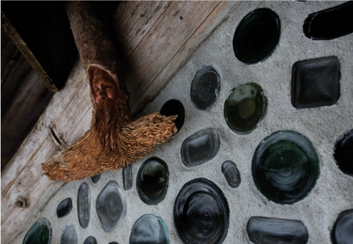
ABOVE: As a symbolic guard of the house, a carving that was given as a gift is on an exterior pantry wall where bottles are cemented into the structure at Donna Kausen's home.
