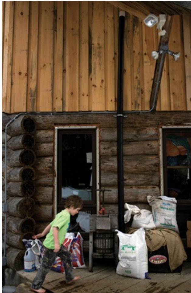
Six-year-old Bazel Russell walks onto the porch at Earthwise Farm and Forest. The black pipe in the center of the photograph leads to the farm's root cellar. Carl Russell said in the summertime, the afternoon sun heats up the pipe, drawing moisture from the cellar.
