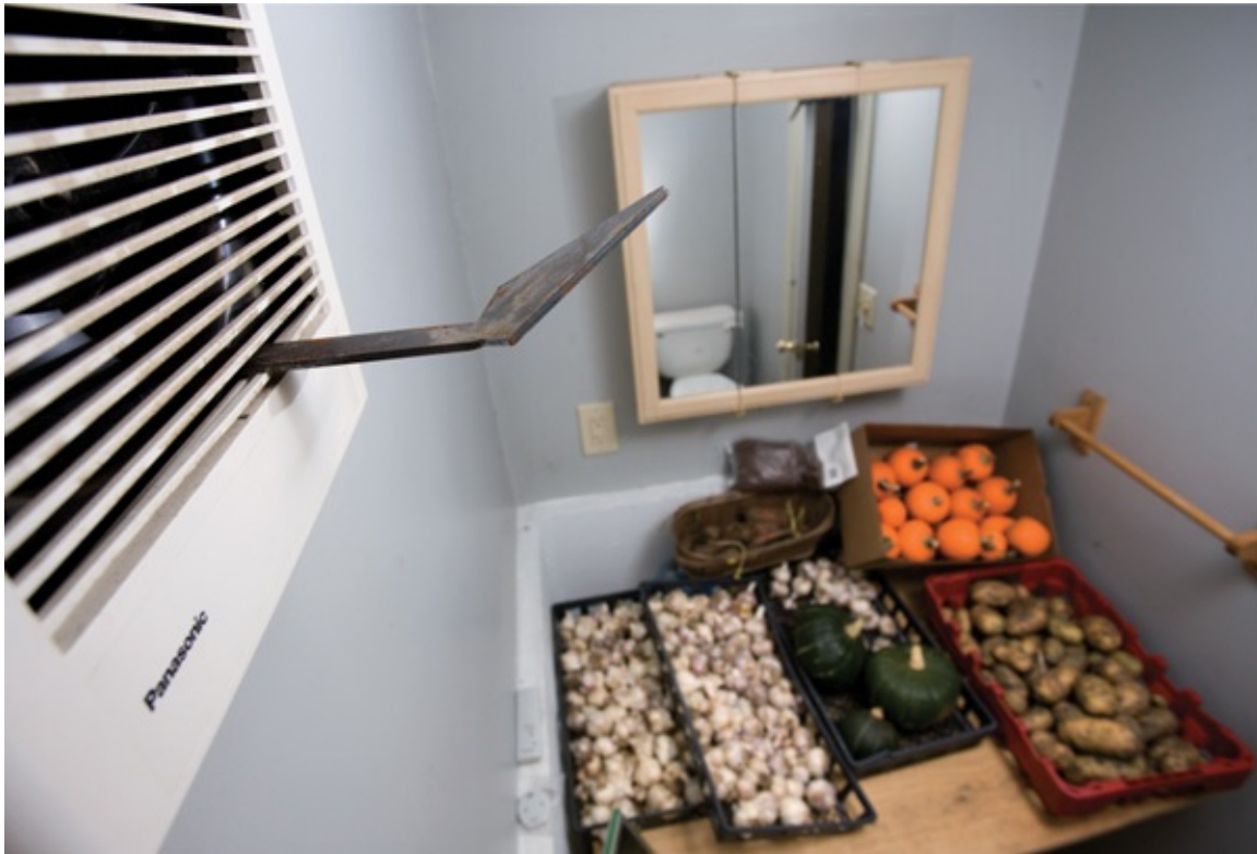
A rod stuck into an old bathroom vent controls the airflow to a cold space in MaryKaye Maxwell's garage. Keeping the room at about 50 degrees, Maxwell stores vegetables from her garden in the space.
